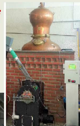
AHP 60 kw ecoHORNET & Alambic (motorina)
