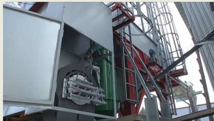
2 x GHP 300 kw, ecoHORNET & Silos Cordoba
