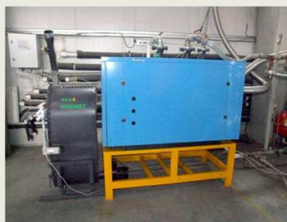
AHP 200 kw ecoHORNET & Buderus (gaz, motorina)
