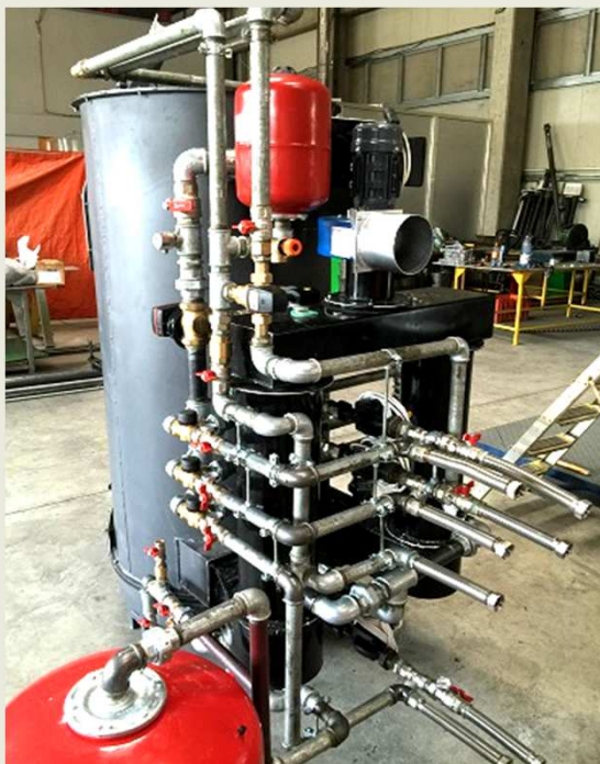
Centrala, puffer, boiler 3 in 1
