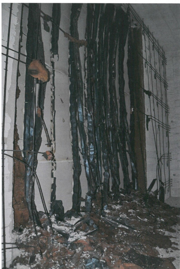
Fig. 8. Exposed side of test specimen after the test
