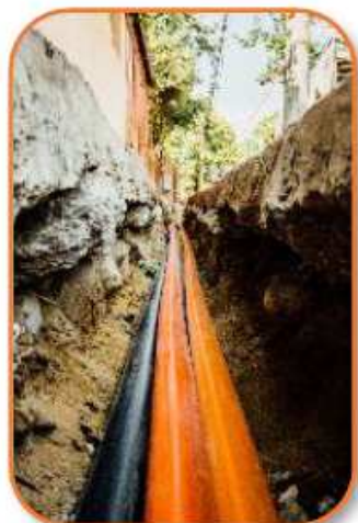
Netcity's underground ducts
